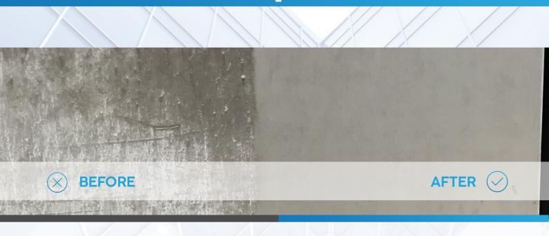
Anodised aluminium also shows signs of aging by fading and oxidisation. Fillers used to clog anodic coating during electrolyse tend to deteriorate with time and expose mill aluminium underneath it. Exposed to weather condition this aluminium will oxidise.
